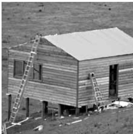
Above left: Colorbond roof, foil backed insulation blanket and polyester batts. Above: Western red cedar cladding to finish.
